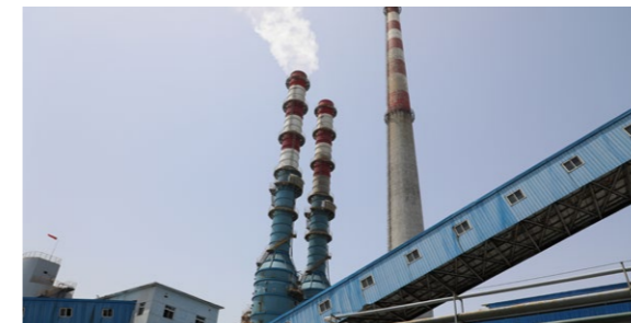
Desulphurization and Denitrification Facility
