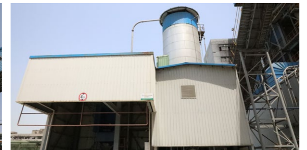
Polymer Denitrification Facility
